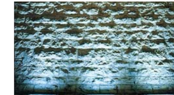
3 recessed LEDline 2 wide beam (BBS 716) Distance wall / optical unit: 250 mm Wall height: 4.5 m
